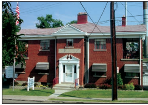
A total of 18,000 sq. ft. of office, shop & showroom space is provided by Pioneer’s Cheviot, Ohio HQ. The sign over the front door reads “Mildred” for Joe (the builder) Westerhaus’ sister.
